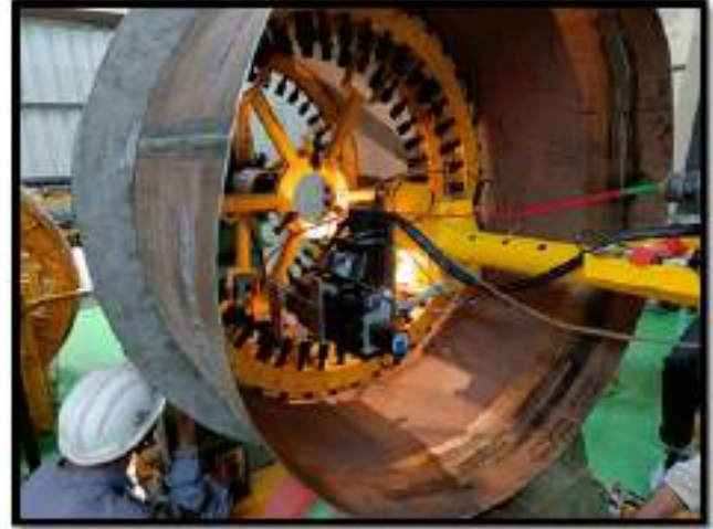
Figure B.2.2: Welding trials to qualify L-seam and C-Seam welding in Integrated Vacuum Vessel.
